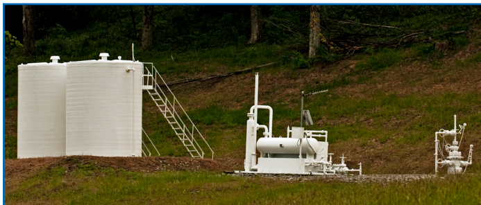
Completed drill site in West Virginia.
